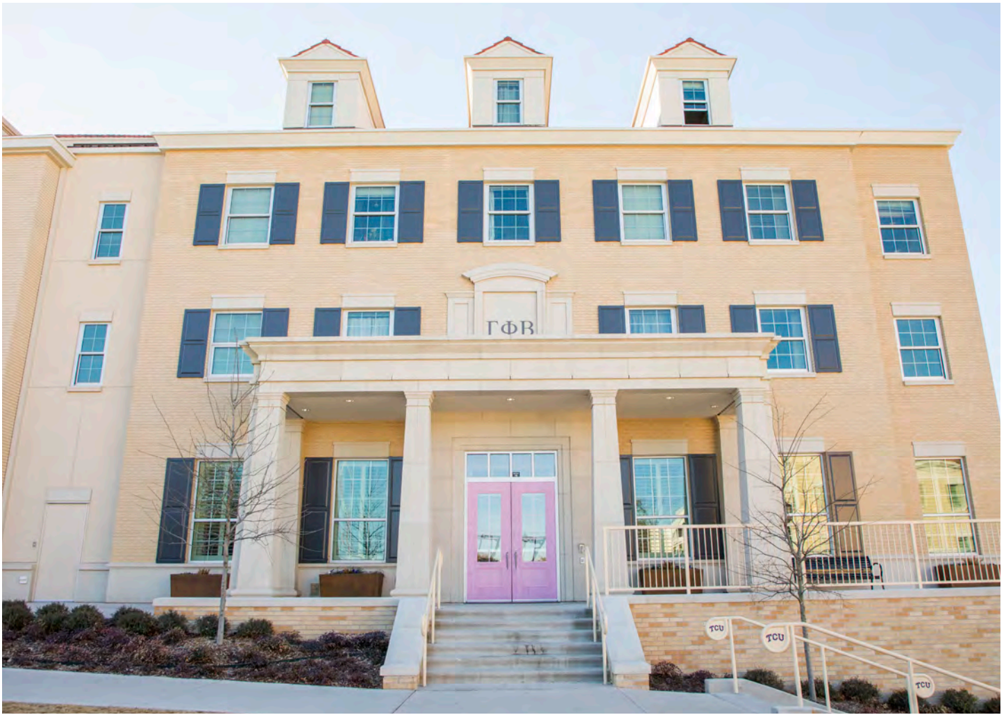
All are welcomed to the Gamma Phi Beta facility by these stunning, pink double front doors.
